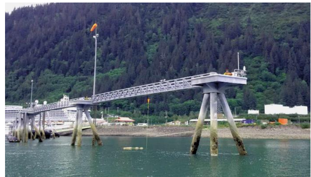
Figure 4 The Nortek 400 kHz 2D Profiler is installed on one of the pilings at the end of the pier. A cruise ship can be seen in the foreground.
