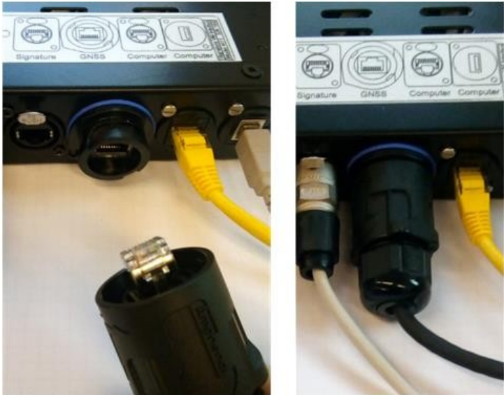
Figure 32: Connecting the GNSS to the Interface Box
